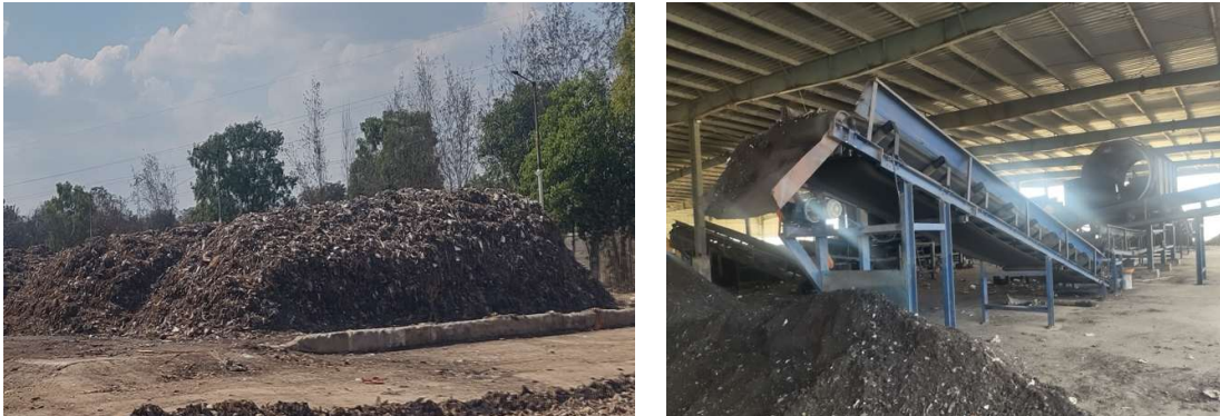
Fig. 3.11 Windrow composting and processing unit
