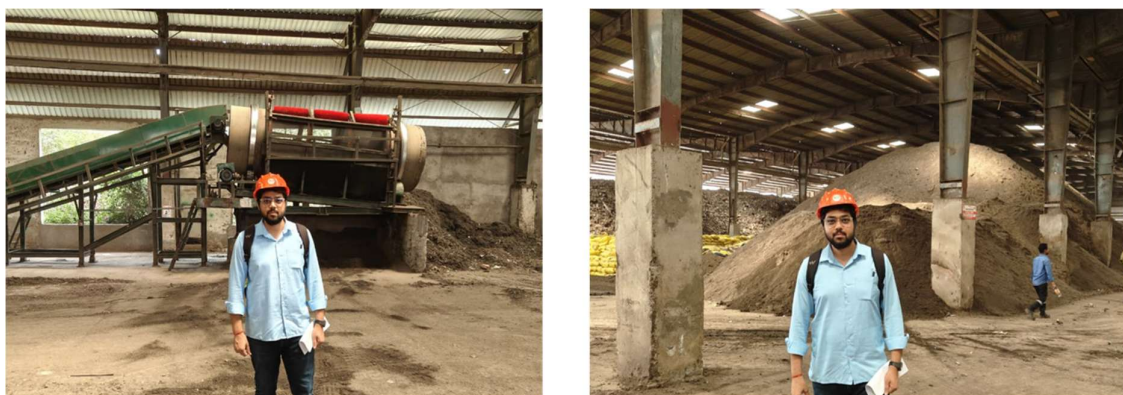
Fig. 3.15 Composting plant at Bawana, New Delhi
