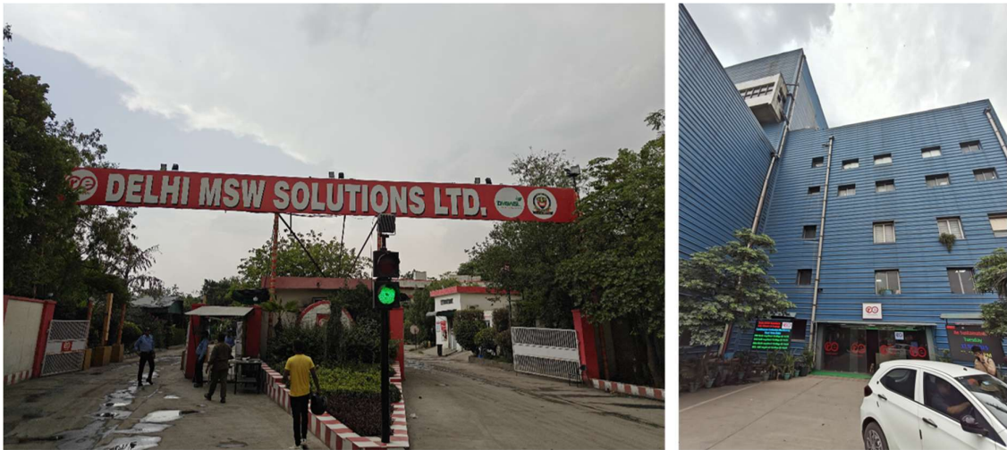
Fig. 3.16 WTE plant at Bawana, New Delhi
