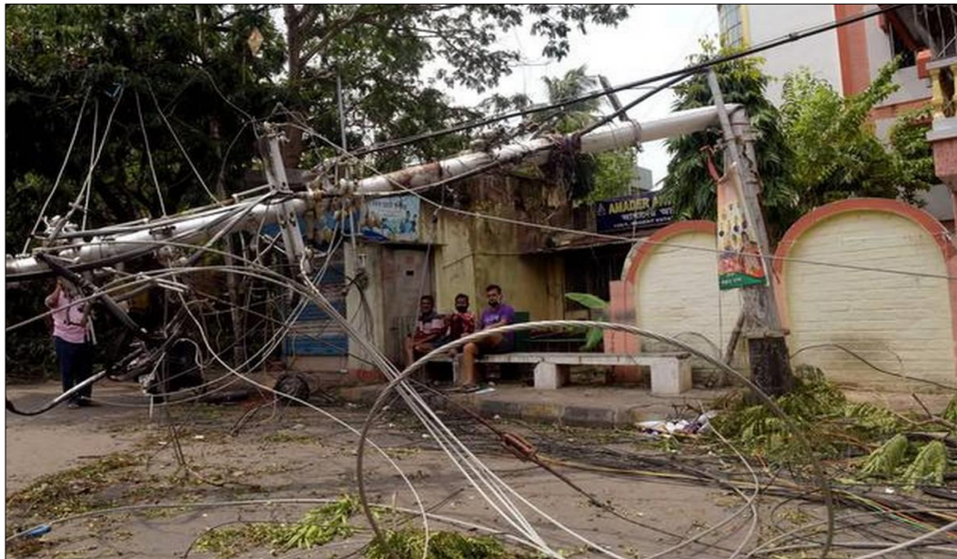
Figure 11: Disruption in Communication lines due to Cyclone Amphan, 2020 16
