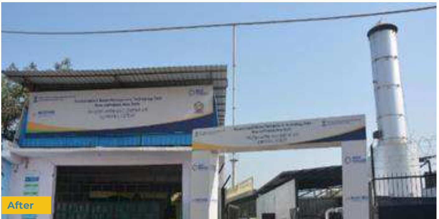
Figure 7: Decentralised Waste Management Technology Park
