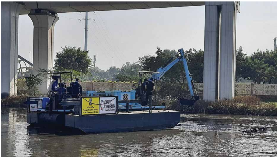
DM-80 installation in Barapullah drain, South Delhi
