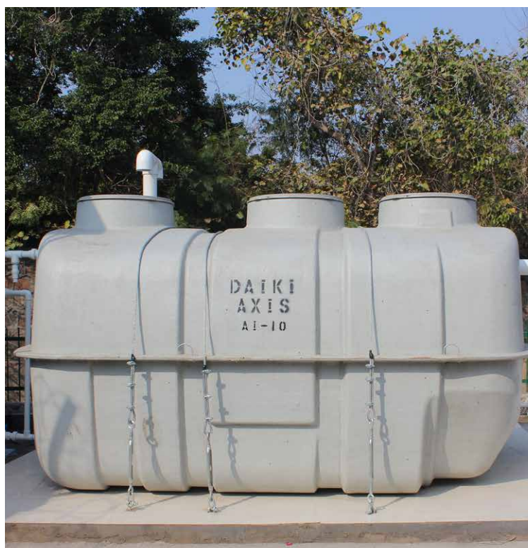
Pilot Installation of Johkhsou Sewage Treatment Plant at Waste to Wealth Technology Park
